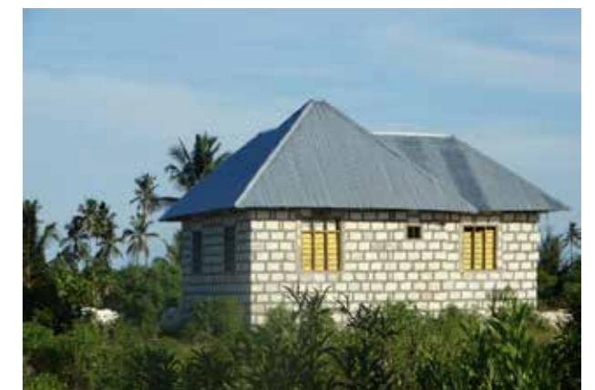
Plate 4. 4: House constructed by limestone bricks and Aluminium sheet roof
