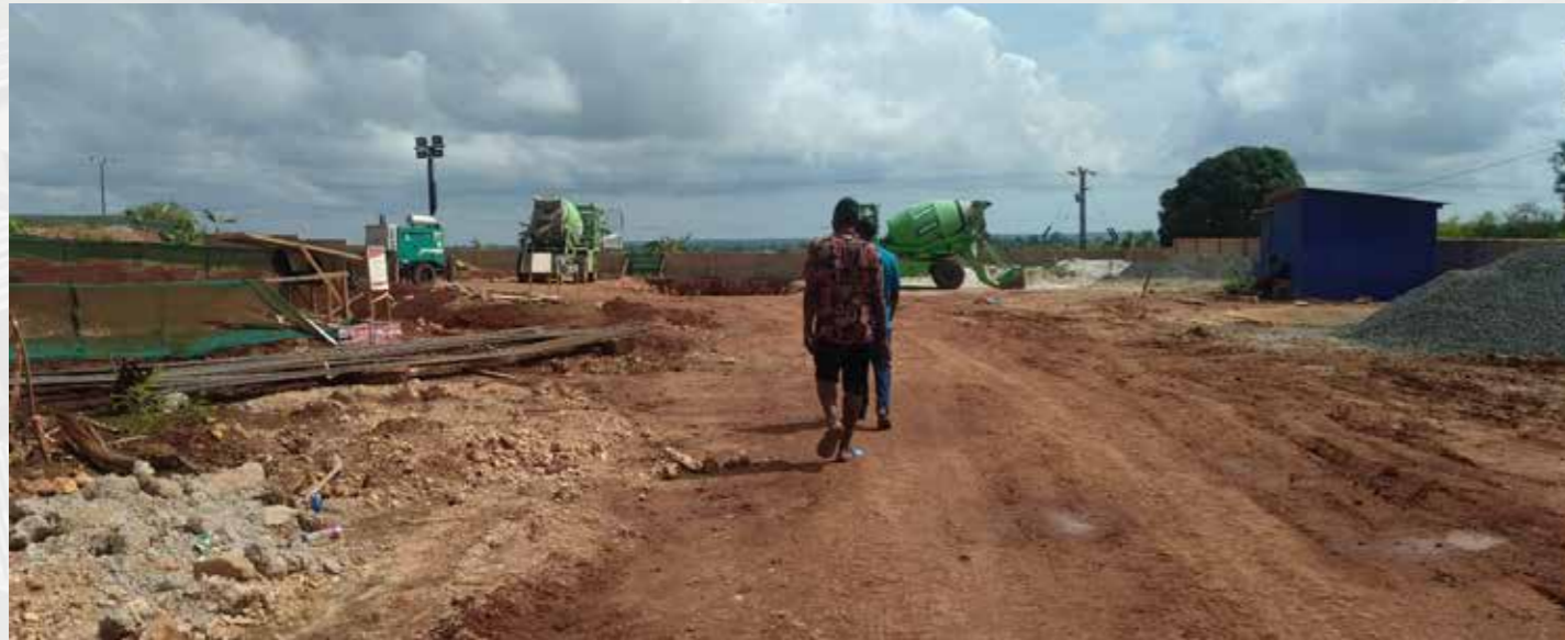
Plate 3.27: Construction site for water storage tanks at Dimani
