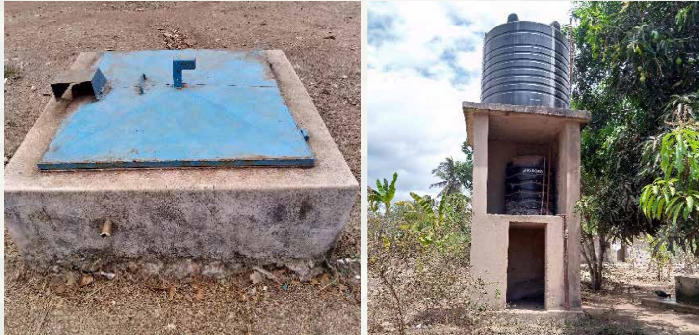
Plate 5. 5: Community well supplying water at Nyamanzi shehia
