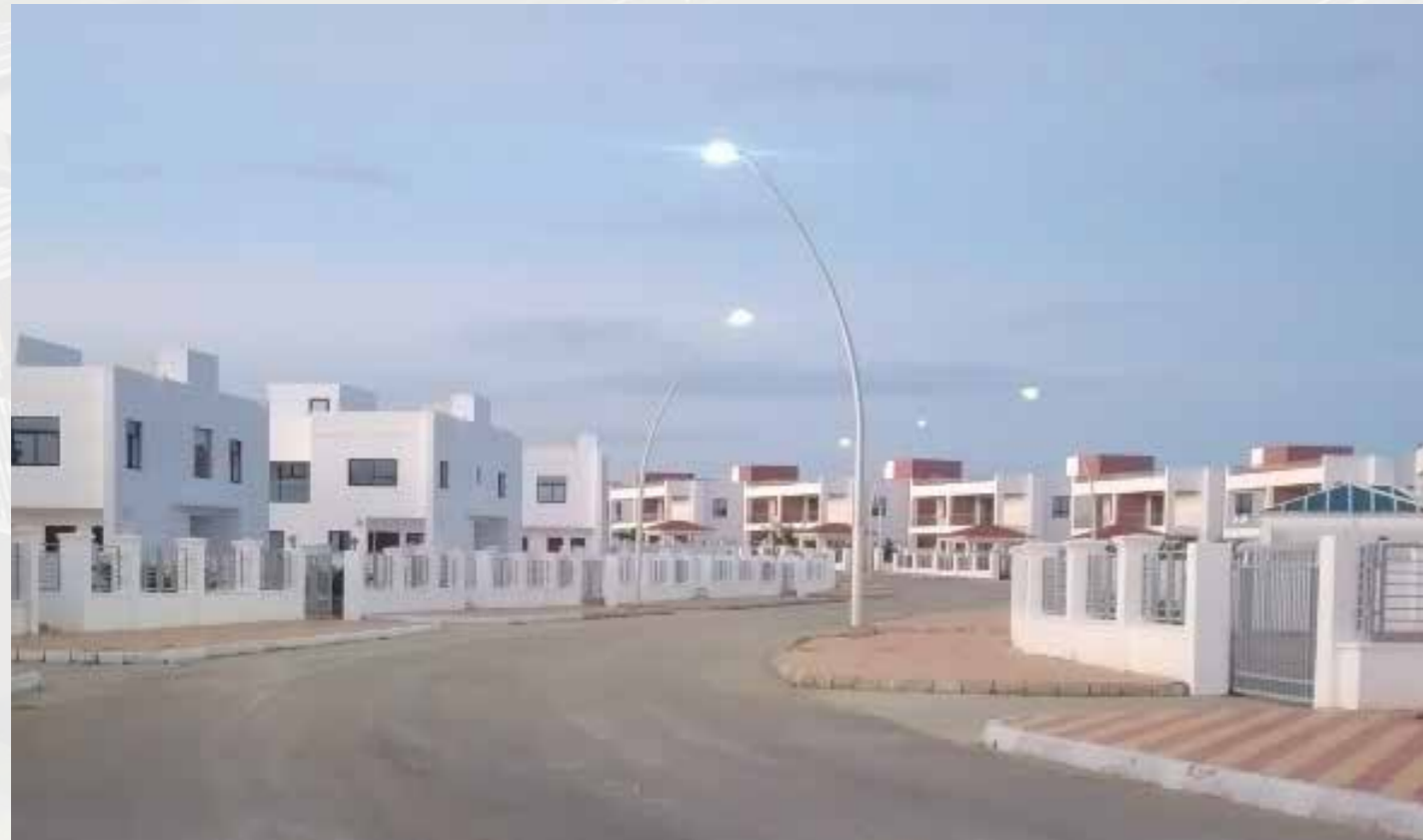
Plate 3. 8: Real Estate Development in Bakhressa Site at Fumba Free Economic Zone
